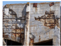
Spalling Due to Corroded Rebar
