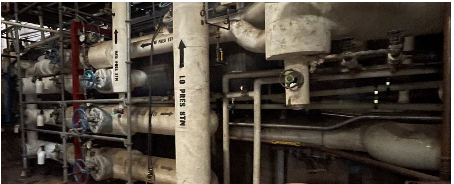
Figure 4: Existing steam infrastructure
