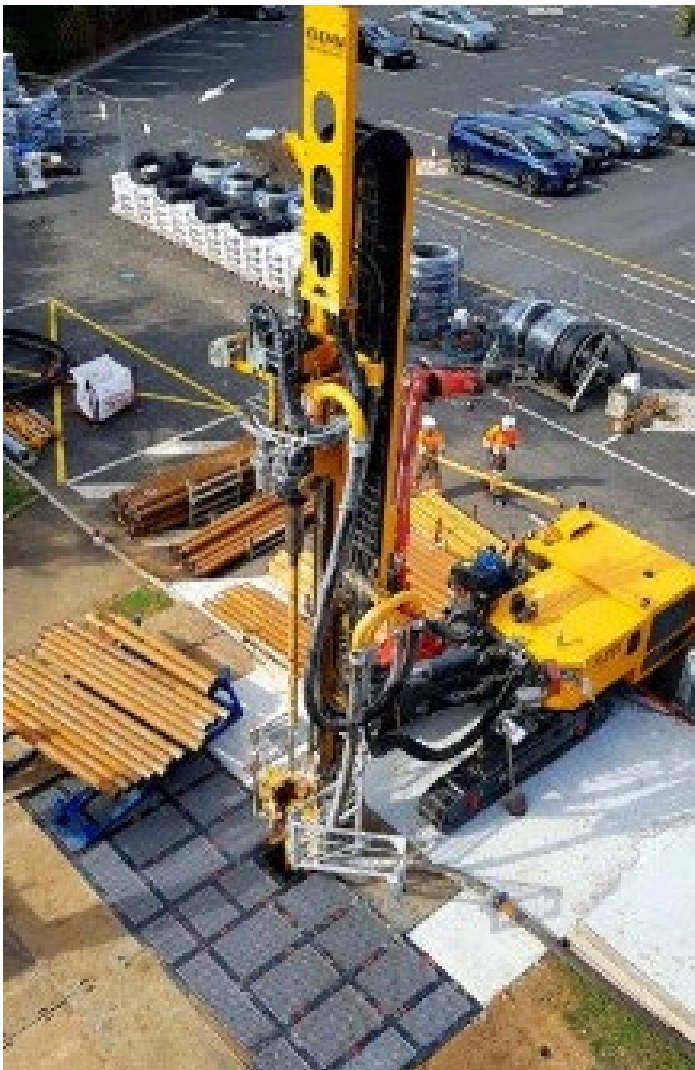
Figure 7: Minimally invasive geothermal well drilling
