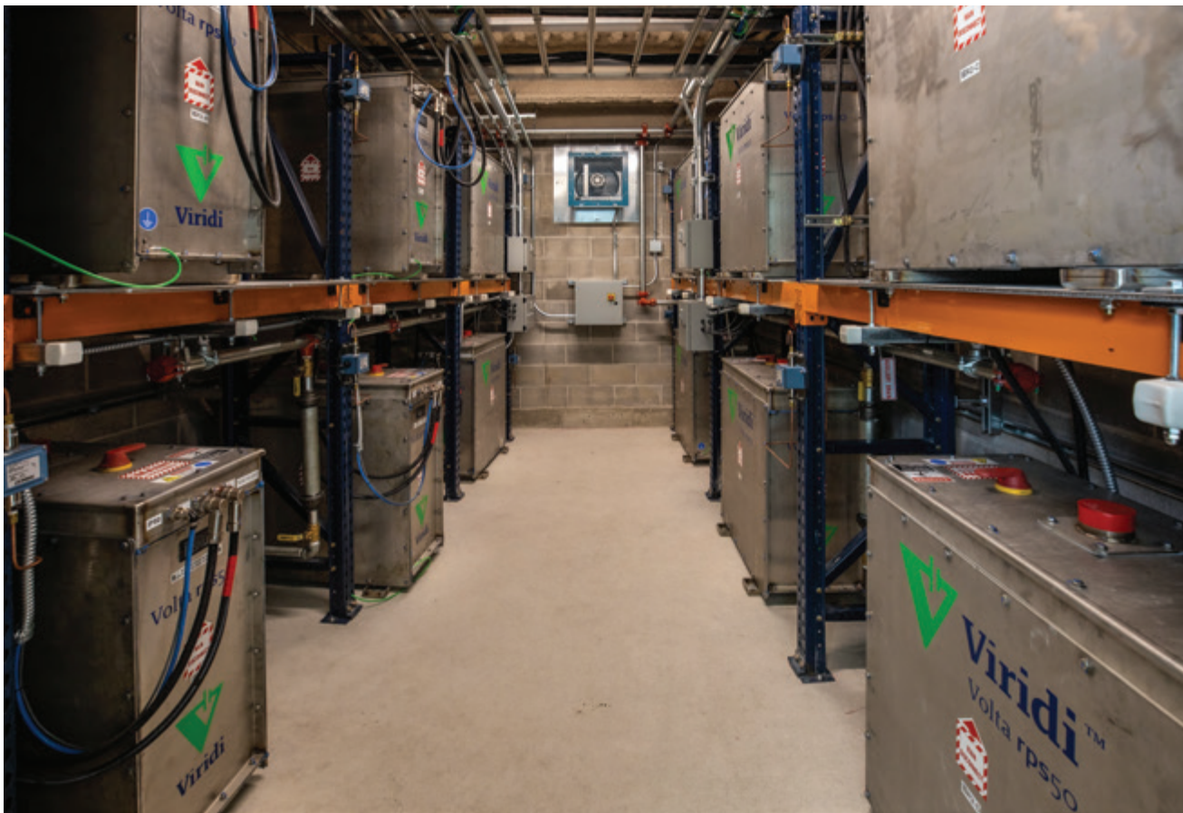
The Battery Energy Storage System (BESS) shown above consists of 12 batteries plus sophisticated control electronics that provide the power storage for the system at HWI.
