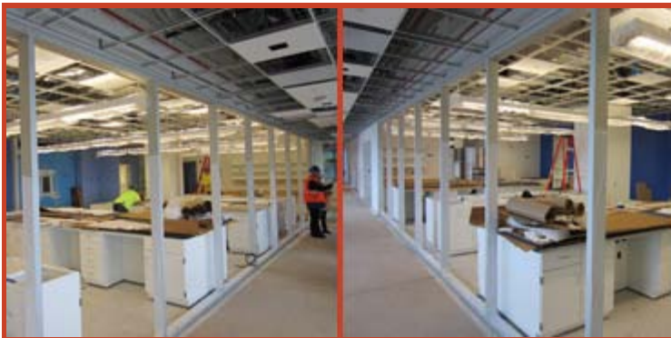
Sixth Floor: Laboratories nearing completion
