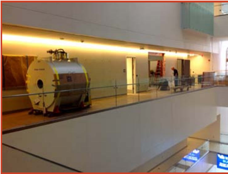
The imager is moved along a reinforced path to its room in the Imaging Center
