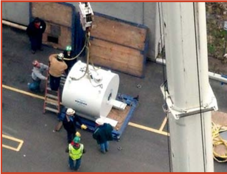
The MRI magnet is being hooked up to a crane
