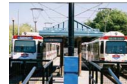
An elevated TRAX station in Salt Lake City
