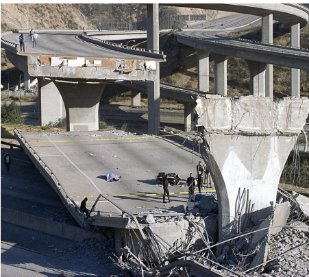
Highway bridge collapse (Sylmar, California, 1994)
