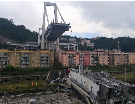
Genoa bridge collapse (Italy, 2018)
